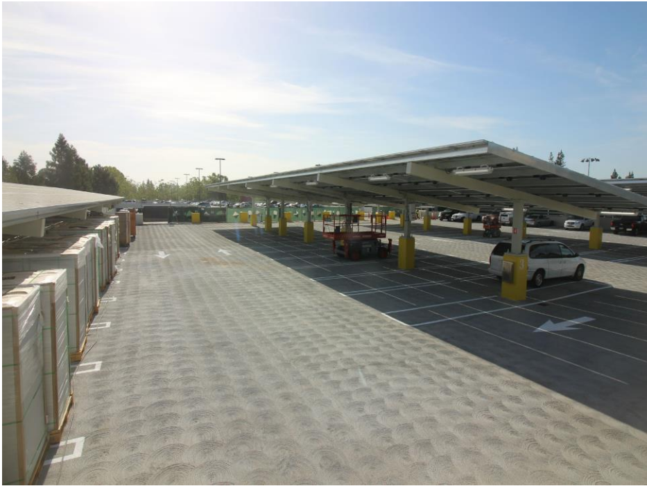
New Garage Expansion Photo Date 05/09/17
