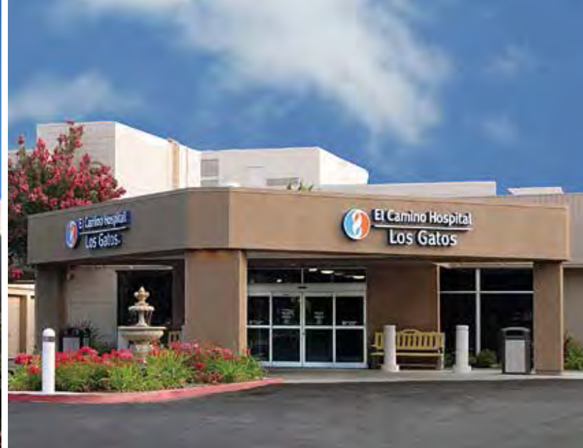
El Camino Hospital, Mountain View
